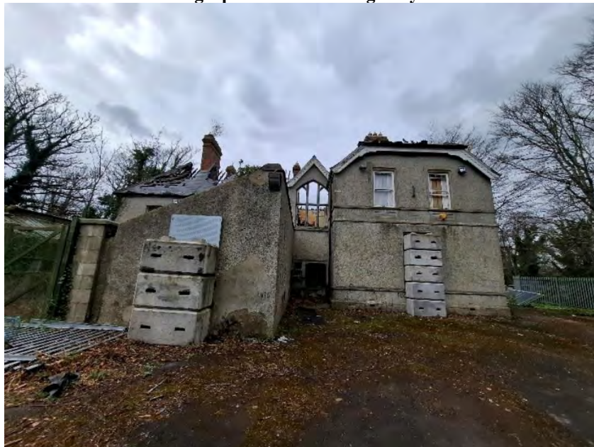
Photograph 3 - Access door closed off.
