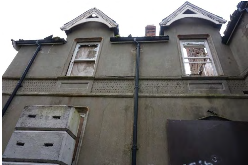
Photograph 23 - Decorative sand cement/OPC reveals and panels.
