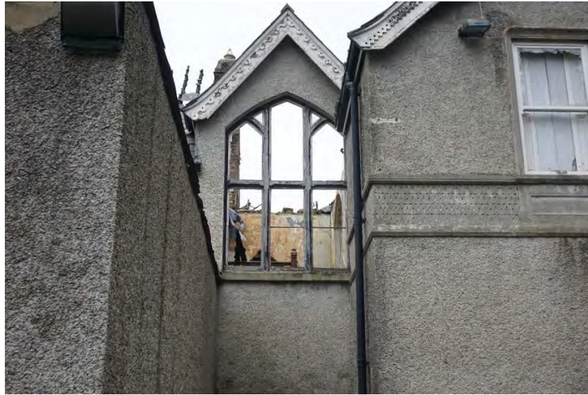
Photograph 4 - Gothic style church-like timber fixed pane window.
