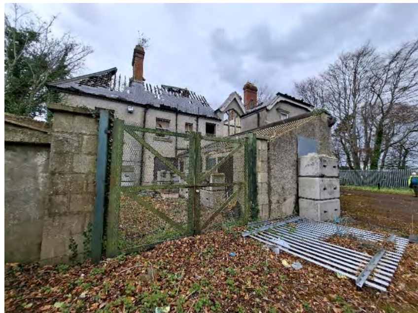
Photograph 5 - Access to southeast facade restricted.
