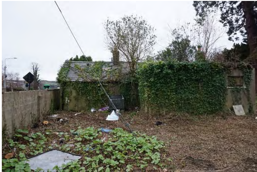
Photograph 22 - Concrete blockwork replacement roadside boundary.
