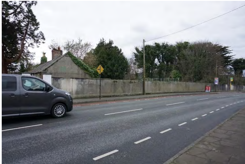
Photograph 20 - Concrete blockwork replacement boundary.
