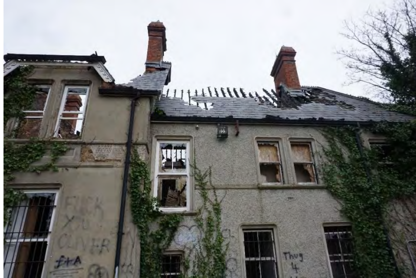
Photograph 25 - Decorative reveals carried over to the double hipped portion.
