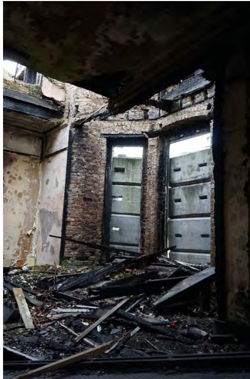
Photograph 10 - Inner face of ground floor bay window.
