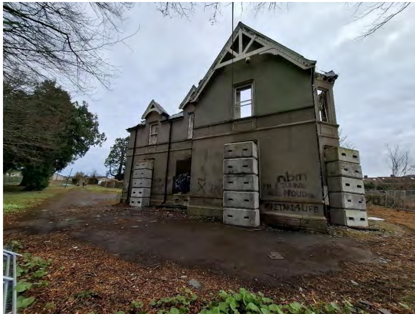
Photograph 7 - Showing the decorative fascia to the roof overhang on projecting gable and dormer windows.
