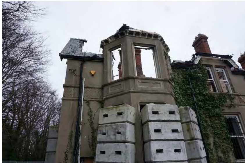
Photograph 24 - Decorative sand cement/OPC reveals and panels.
